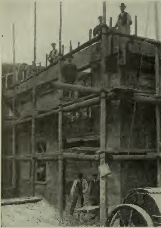
FOOD STORE ON LORD ASTOR'S FARM, COOKHAM, BERKS : DURING CONSTRUCTION.
